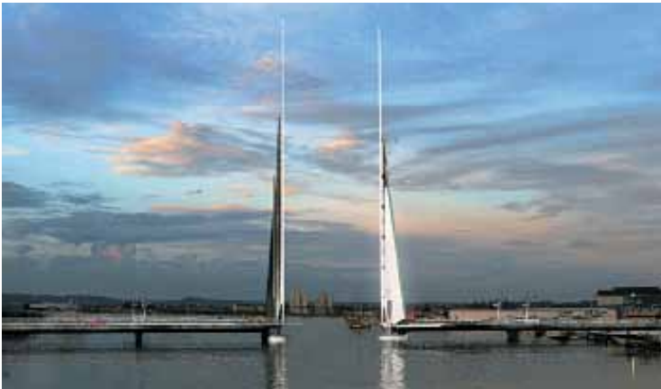
← Twin Sails Bridge now under construction
